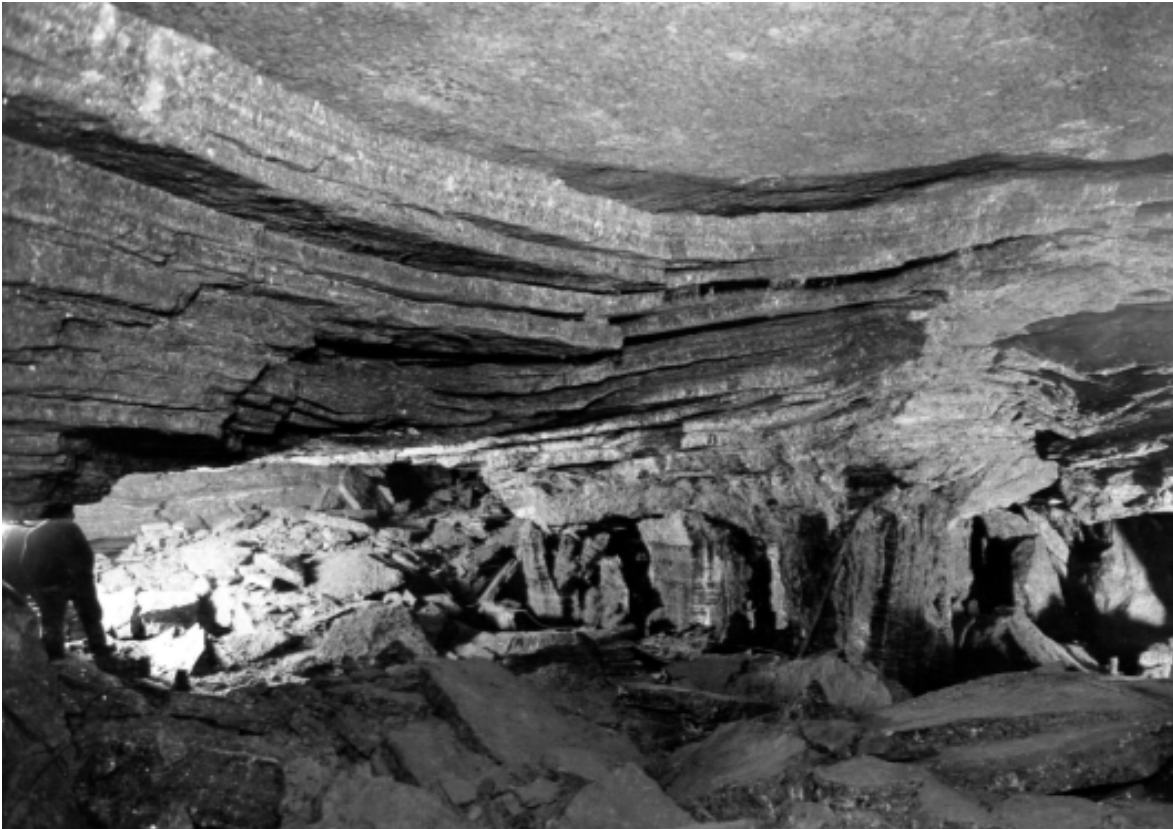
Figure 3 - Roof and pillar close to the external abutment in the collapsed Saint-Maximilien panel (CSME Archives).
