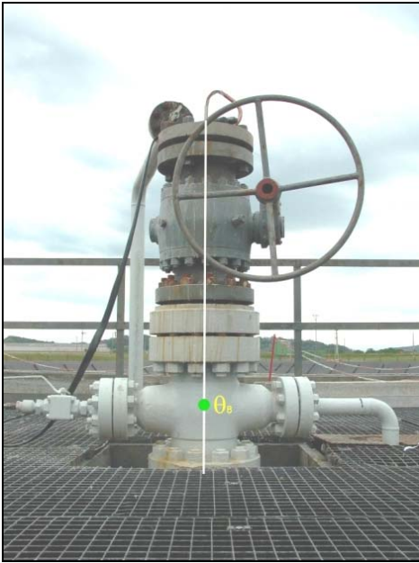
Picture 4 – SPR3 wellhead and \theta_8 gauge location.
