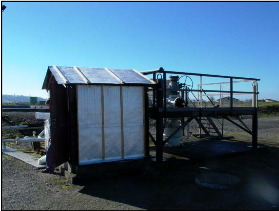
Picture 1 – Hut enclosing data recording devices close to the wellhead.
